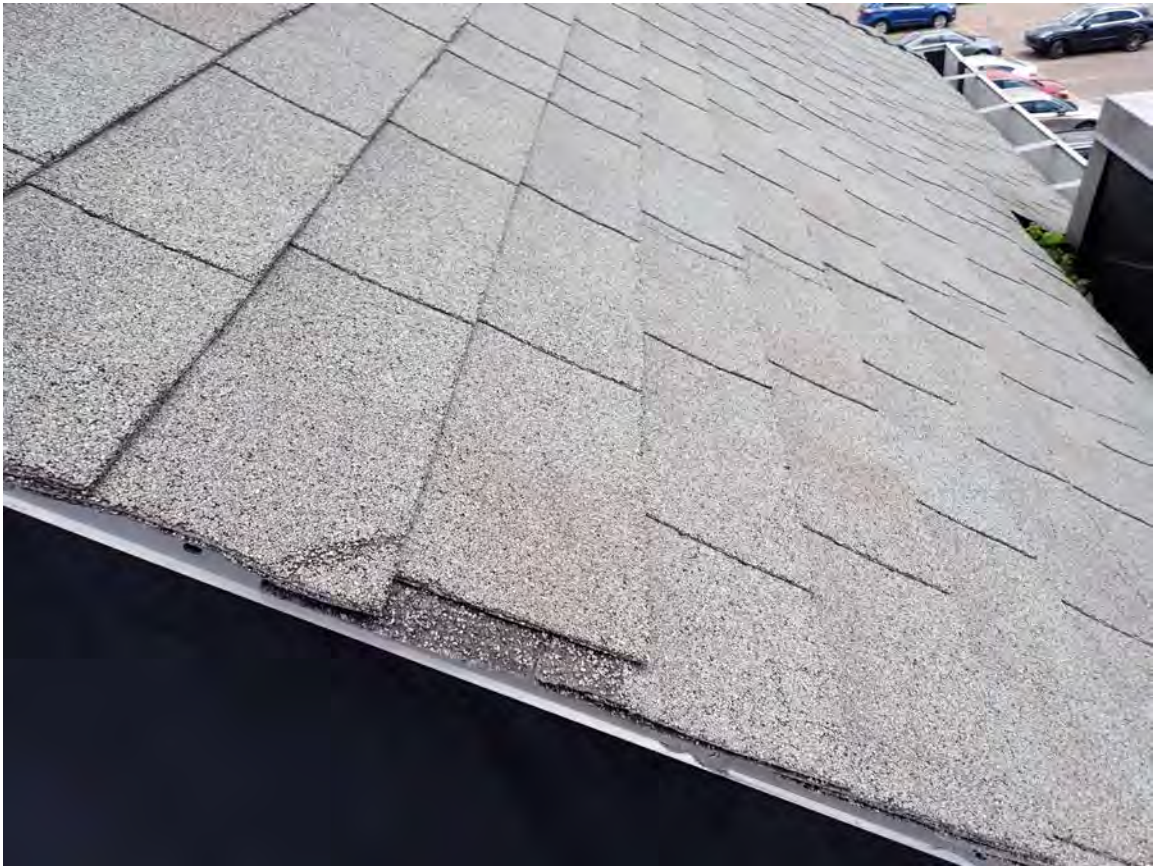
Existing Kroger Store D-442 Roof – East Side Asphalt Roofing Shingles and Underlayment No Asbestos Detected
