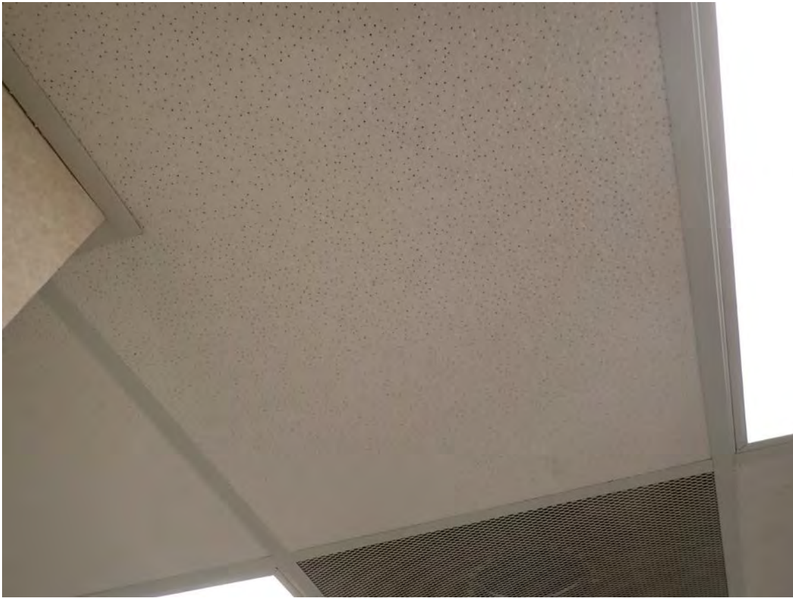
Existing Kroger Store D-442 Office Areas 2' x 4' Acoustical Ceiling Tile (pinhole pattern) No Asbestos Detected
