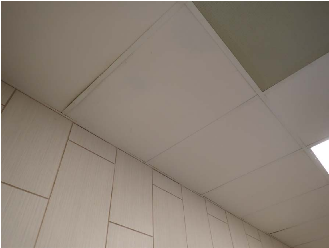
Existing Kroger Store D-442 Food Prep Areas 2' x 4' Acoustical Ceiling Tile (drywall pattern) No Asbestos Detected
