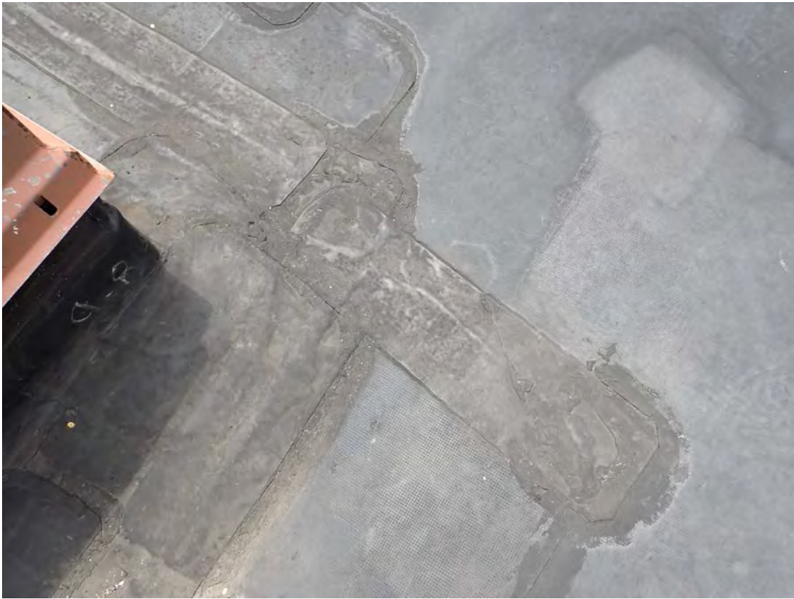
Existing Kroger Store D-442 Main Roof Rubber Membrane Roof Seam Caulk No Asbestos Detected
