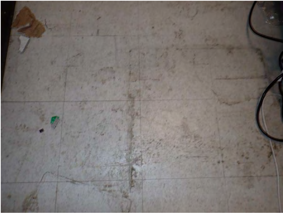
Existing Kroger Store D-442 ECR 12" x 12" White Scale Pattern Floor Tile and Mastic No Asbestos Detected
