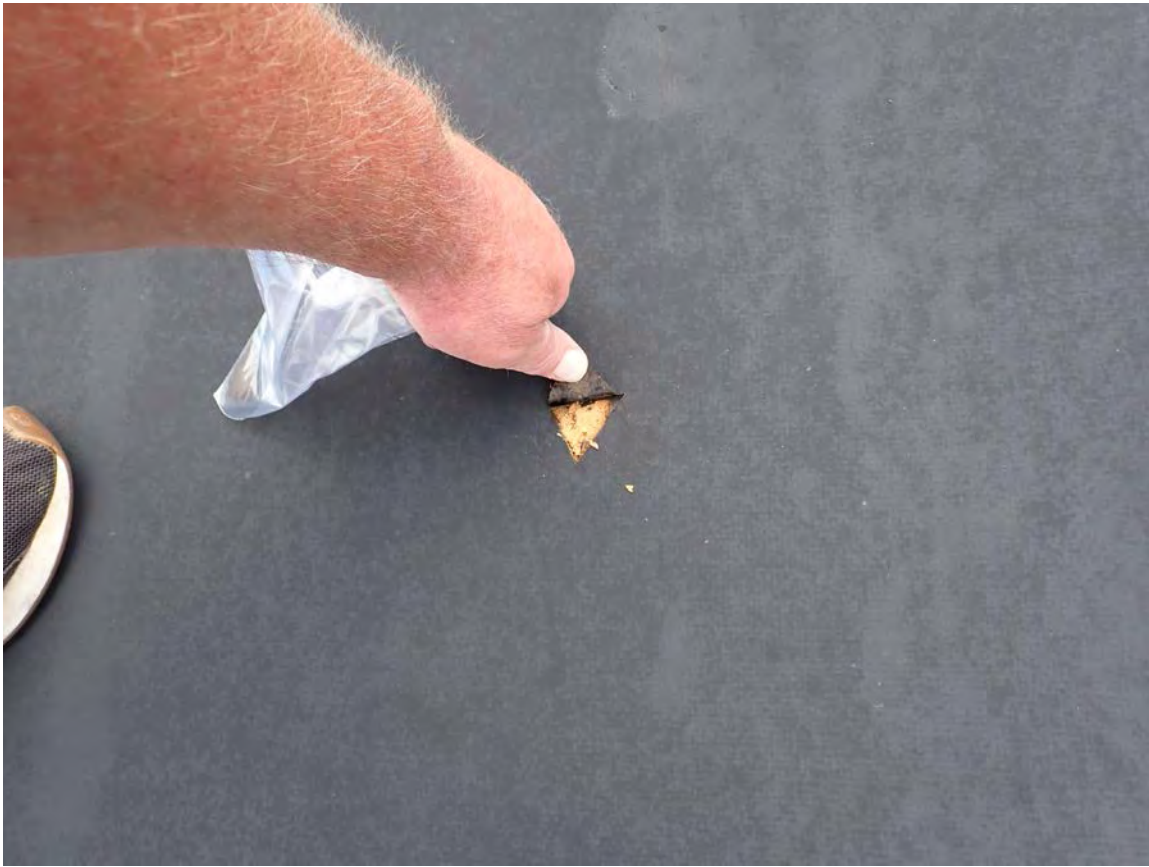
Existing Kroger Store D-442 Main Roof Roofing Felt under Rubber Membrane Roof No Asbestos Detected
