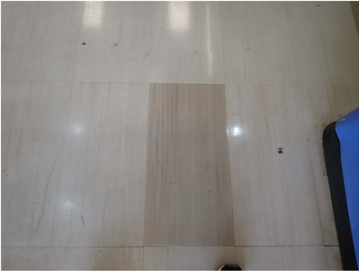
Existing Kroger Store D-442 Store Floor 12" x 24" Tan and Brown Floor Tile and Mastic No Asbestos Detected
